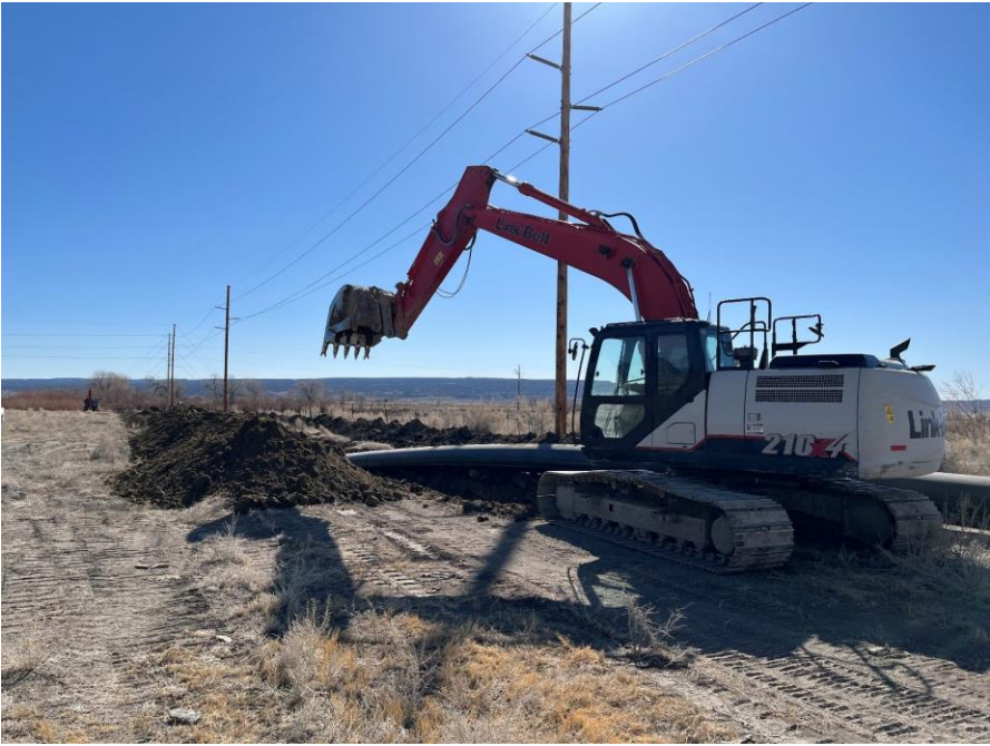
FIGURE 17. Muddy Creek Project
