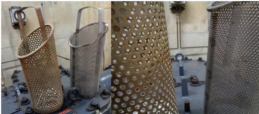
FIGURE 11. Both the old (left) and new (right) strainer baskets sit on top of the housing that they are placed in at Glen Canyon Dam. Behind the baskets mounted on the wall is a glimpse the UV light system.
