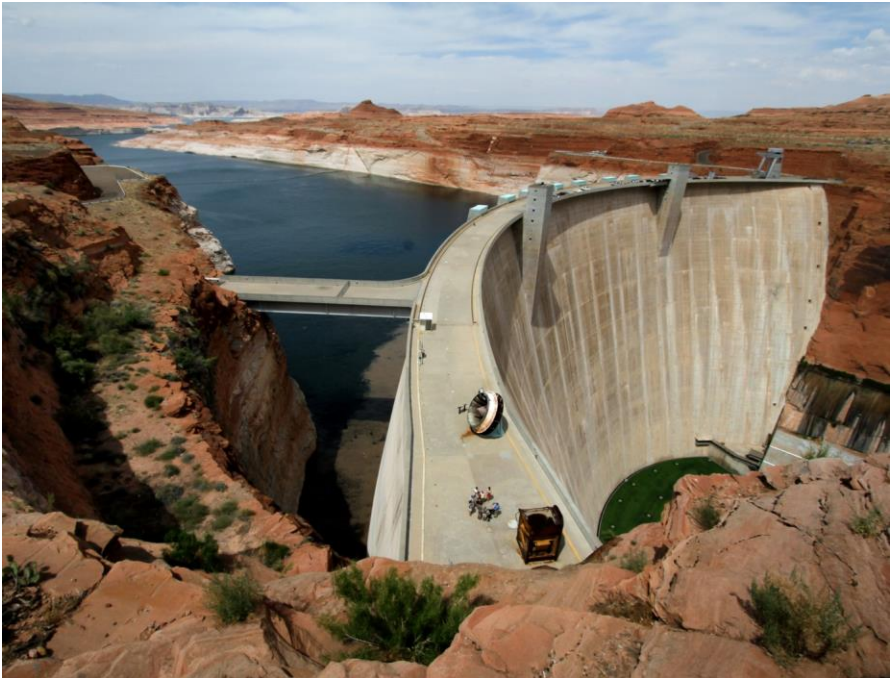
FIGURE 6. Glen Canyon Dam and Low Lake Powell Elevations
